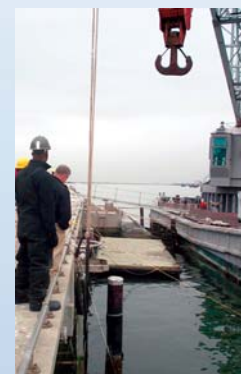
200-ton floating crane preparing to pull a bundle of sensor cables. Photo by UTI (SCW/DV) Martin Stacy.
