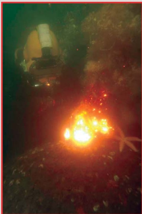
A Diver uses an exothermic cutting torch to remove interference from J-484's external hull.
